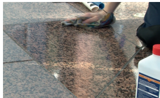
2. CLEAN THE SURFACE
